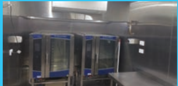
2 x 10 tray combi steamers, a 20 tray blast freezer, and a preparation bench top
